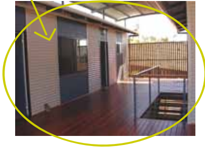
Figure 13 This home has a breezeway between the sleeping and living areas which allows for plenty of air circulation (Photo: ecoSAVVY).
