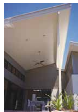
Figure 4 An outdoor area with large openings and access to prevailing breezes (Photo: ecoSAVVY).
